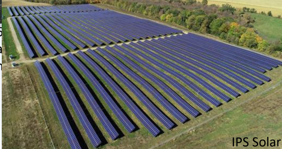
Northfield Area Solar Garden (Northfield MN)
