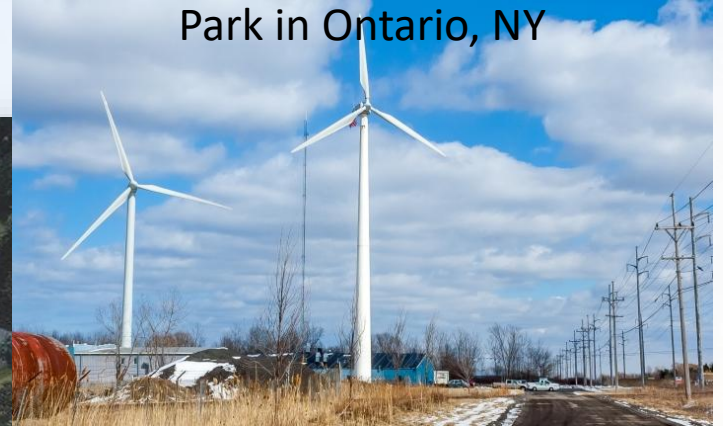
250 kW & 850 kW wind turbines
